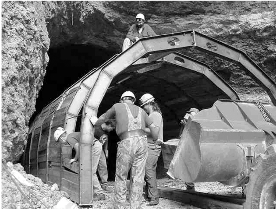
Figure 1. Stabilization arch constructed at Magazine Mine, Alexander County, IL.
