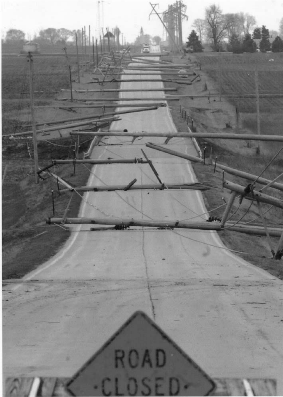
Figure 2. A country road near Mt. Pulaski with many power poles downed by a tornado on March 12. (Photo courtesy of Decatur Herald and Review, and taken by Kelly Huff).
